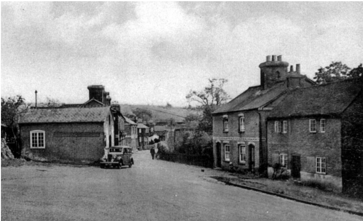
The Chapel & Nos. 21,23 and 25 Lemsford Village, 1936
